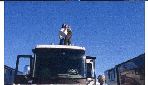
Installing a satellite receiver
